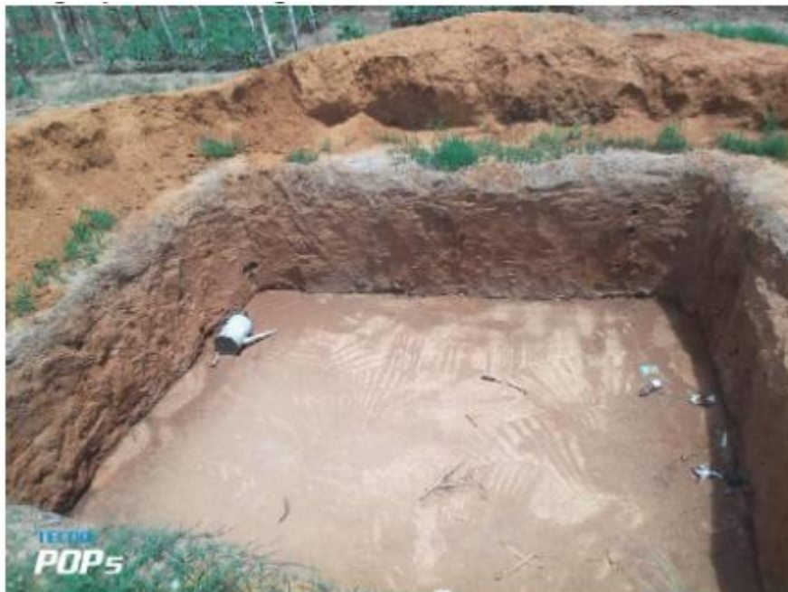
Construction of water troughs
