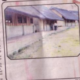
*PART of the Mpongwe Skills Centre structures.
