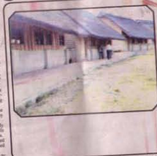
*PART of the Mpongwe Skills Centre structures.
