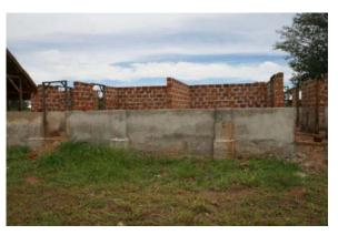
**17 Boarding Boys 1.** Finished interior masonry up to ring beam level including reinforcement of the foundation( $\uparrow$ ).
